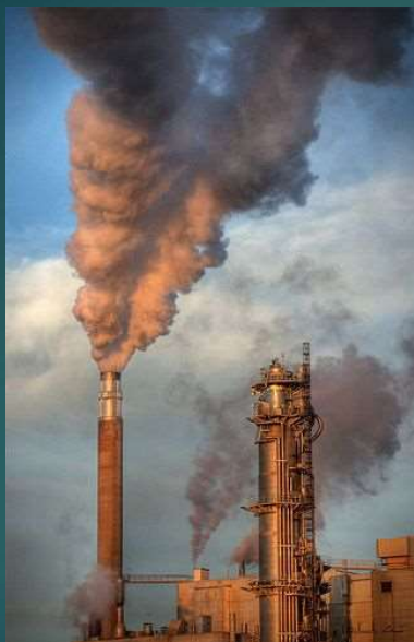
Chemical factory, Poland
